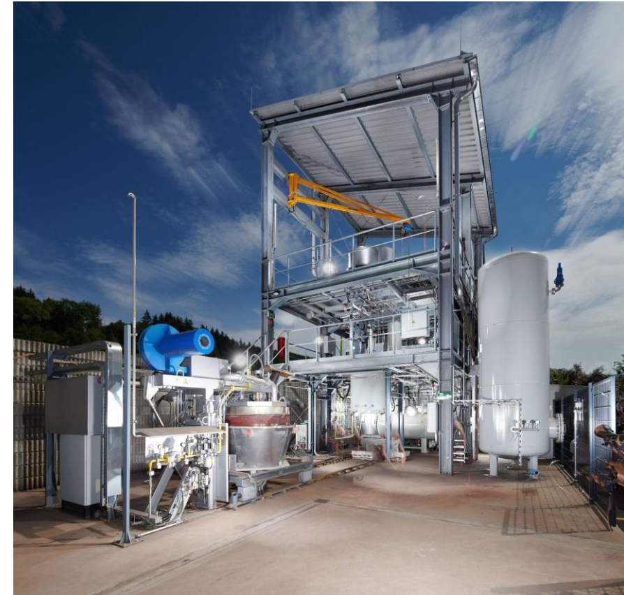
HPSR pilot plant at voestalpine Donawitz site
